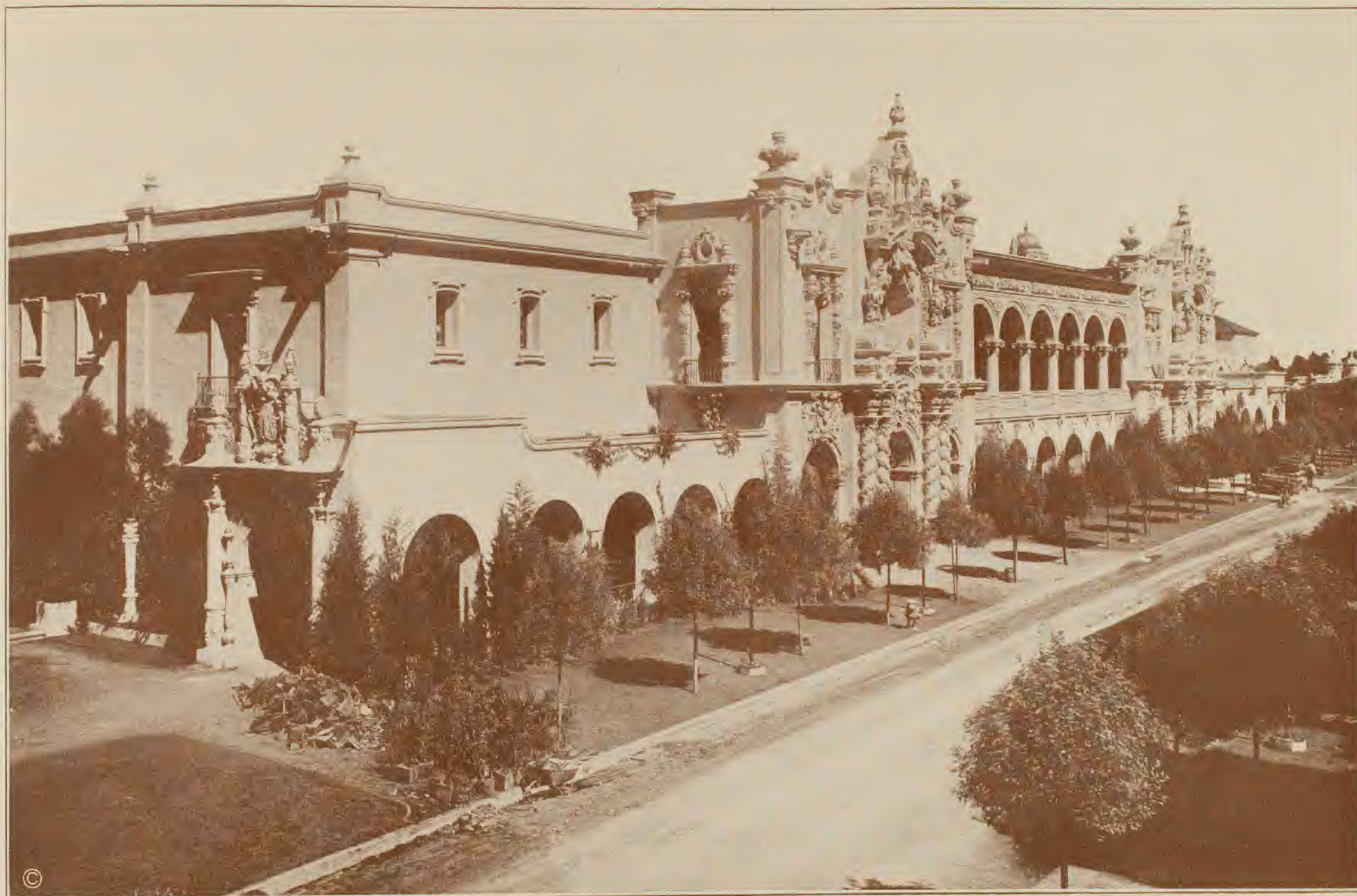
Varied Industries Building, from across El Prado—San Diego Exposition. Photo Supplied by Underwood & Underwood, N. Y.
