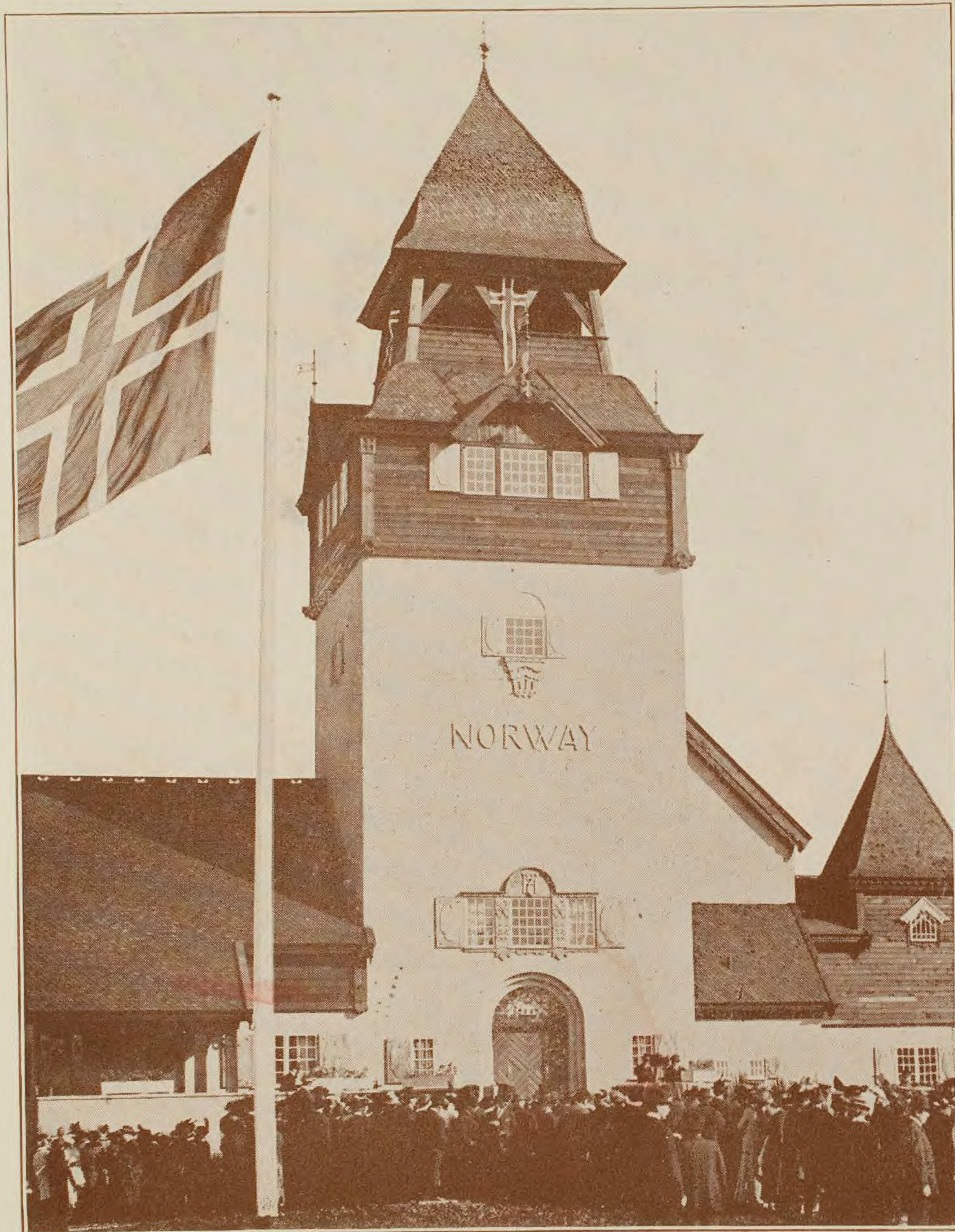
Norway Building, showing dedication ceremonies.
