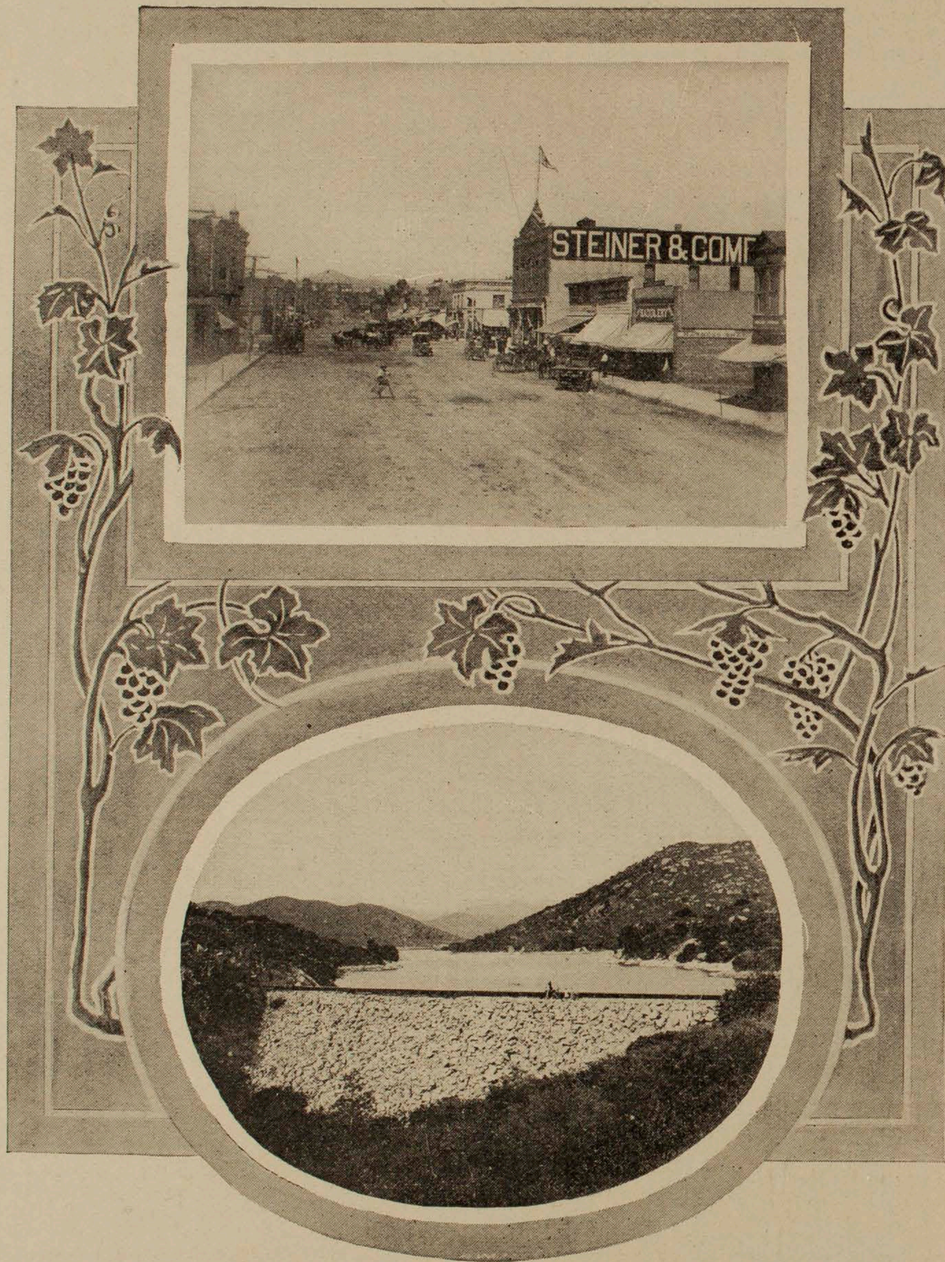
ESCONDIDO STREET SCENE AND DAM
