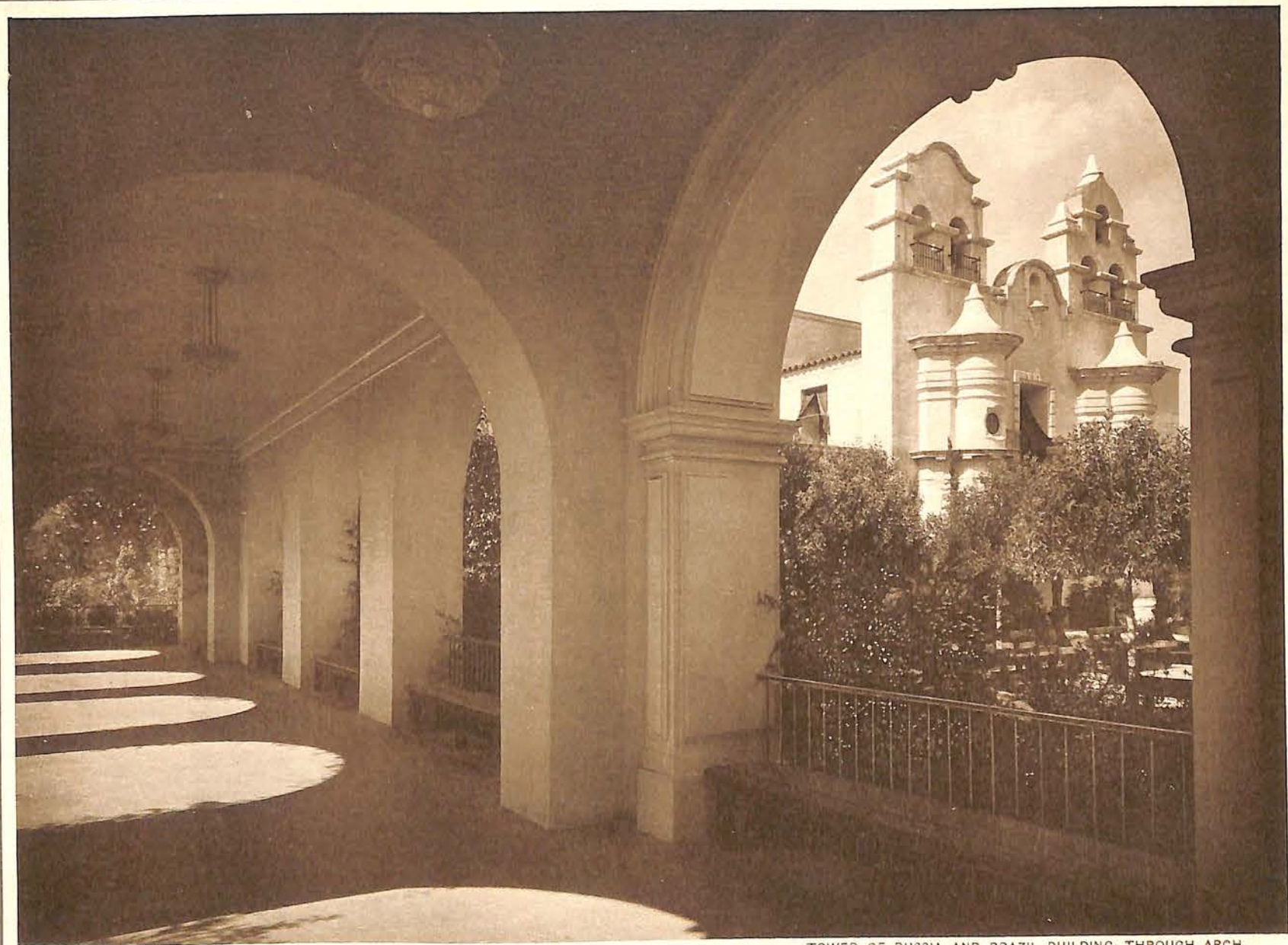
TOWER OF RUSSIA AND BRAZIL BUILDING, THROUGH ARCH.
