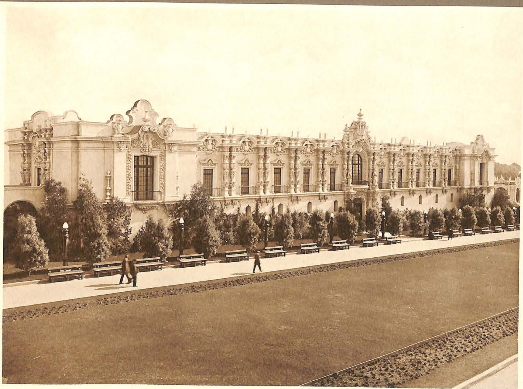
SAN JOAQUIN VALLEY BUILDING.
