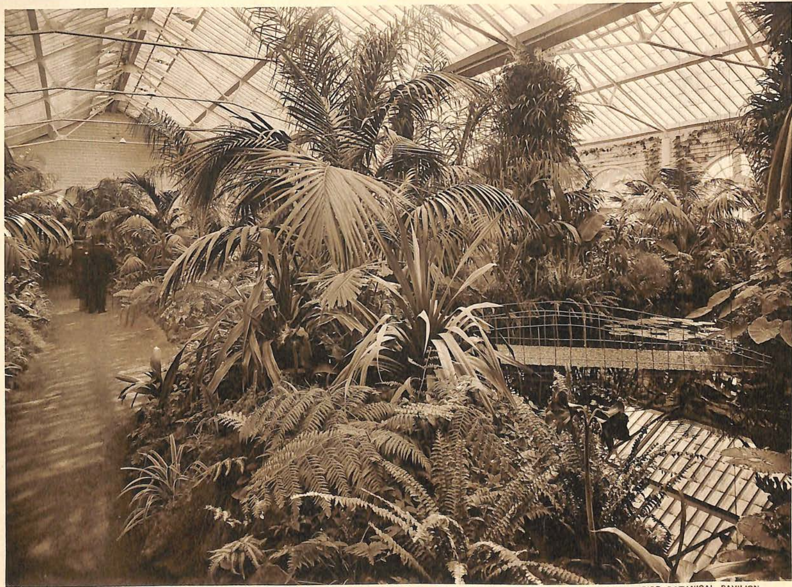
INTERIOR BOTANICAL PAVILION.
