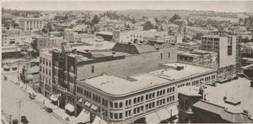
SAME VIEW IN 1911, EXPOSITION SITE IN DISTANCE
