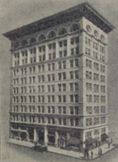
AMERICAN NATIONAL BANK BLDG.
