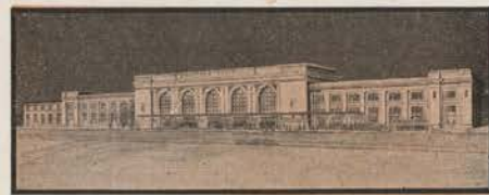
Southern Pacific Station, Los Angeles
