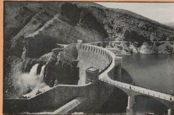
ROOSEVELT DAM, ARIZONA
