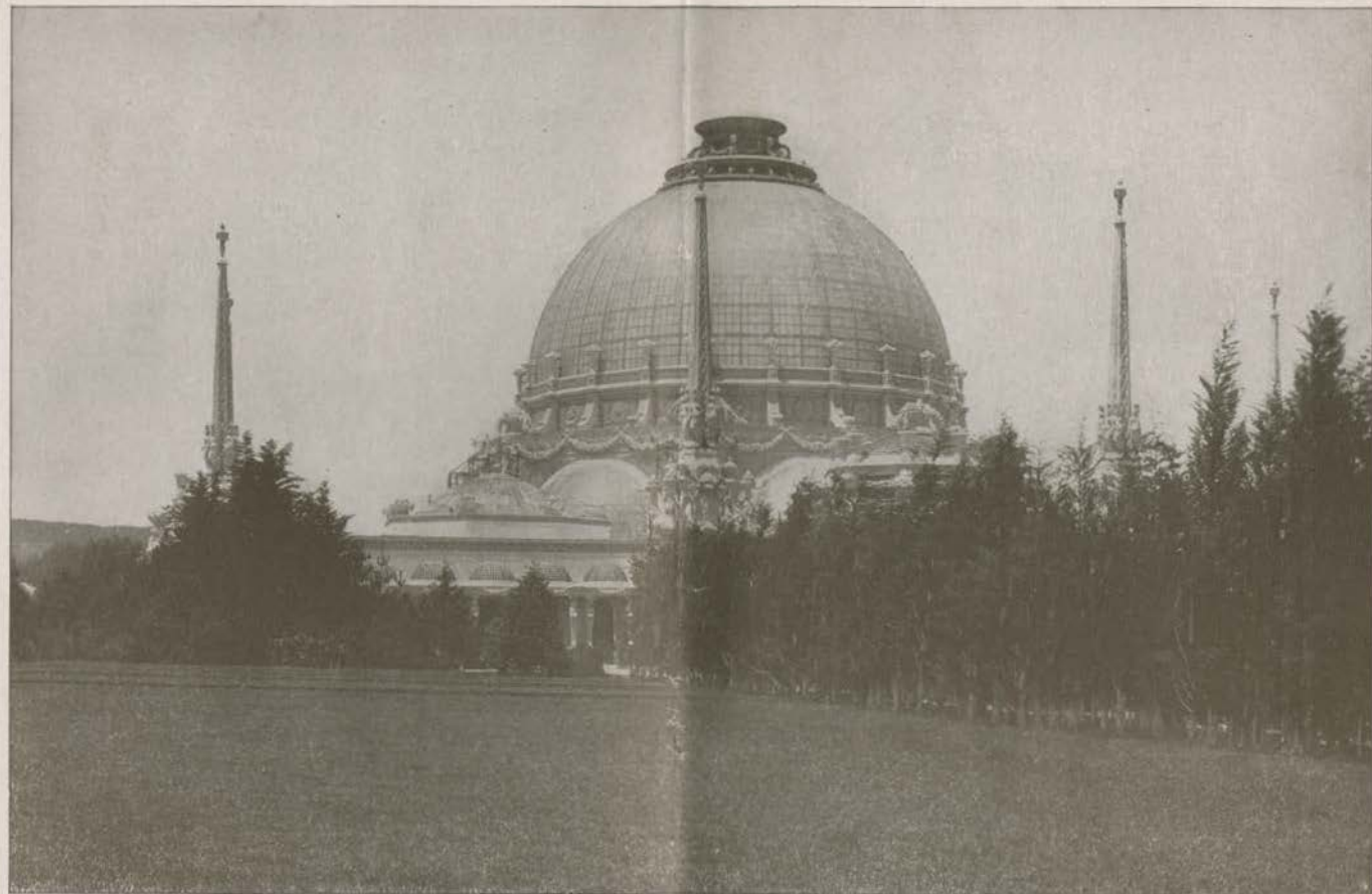
The Glass Dome of the Palace of Horticulture, Largest Hemispherical Dome in the World, 185.5 Feet in Height and 152 Feet in Diameter
