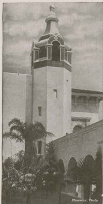
Tower of the Science and Education Building
