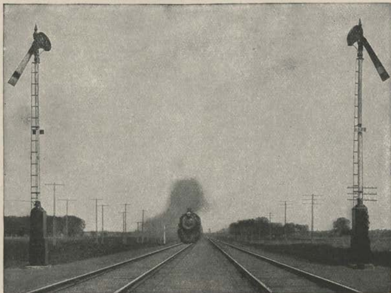
"Safety First!" Every mile of the Union Pacific is protected by Automatic Electric Block Safety Signals to Control Movement of Trains.
