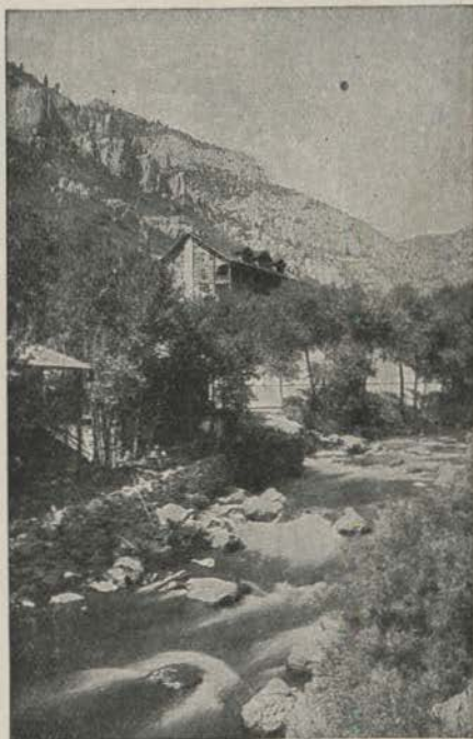
"The Hermitage" seven miles from Ogden, is the oldest Resort in the 15-mile canyon which is included in the City's Boulevard System.
