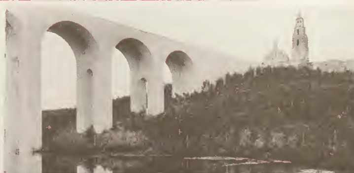
The great Puento Cabrillo, a concrete viaduct spanning Cabrillo Canon, 136 feet below which has been transformed into a beautiful artificial lake.
