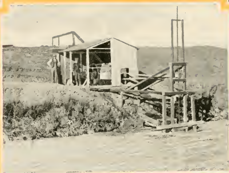
An Oil Engine Pumping Water for Irrigation
