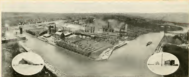
Steel Mills, South Chicago, U S A
