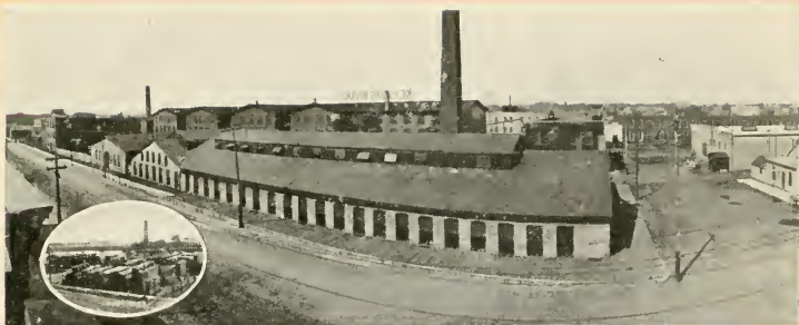
Keystone Works, Rock Falls, Ill., U S A
