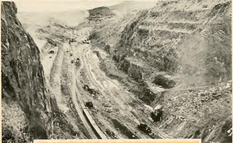
Digging Gaillard (Culebra) Cut
