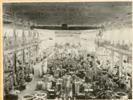
Assembling Room in one of the Engine Works
