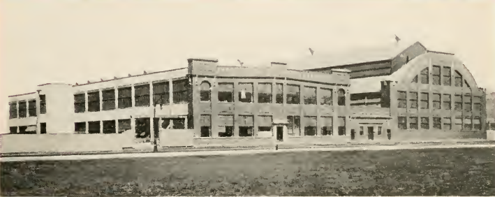
Tractor Works, Chicago, U S A
