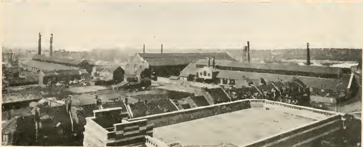
Croix Works, Croix, France
