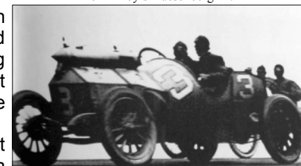
The Tahis Special #3, with its oil cooler on the hood.
