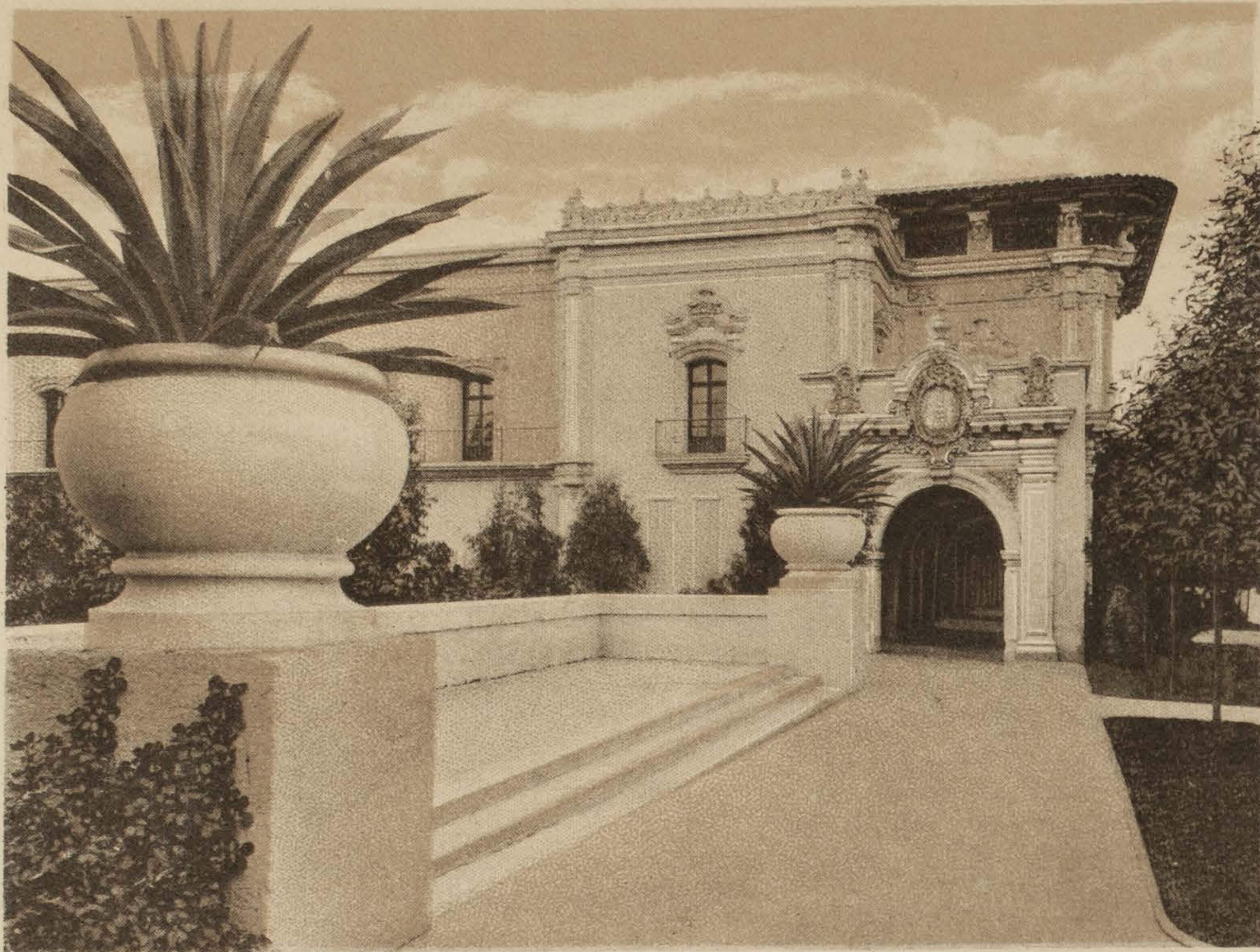
Vista of Commerce and Industries Building.
