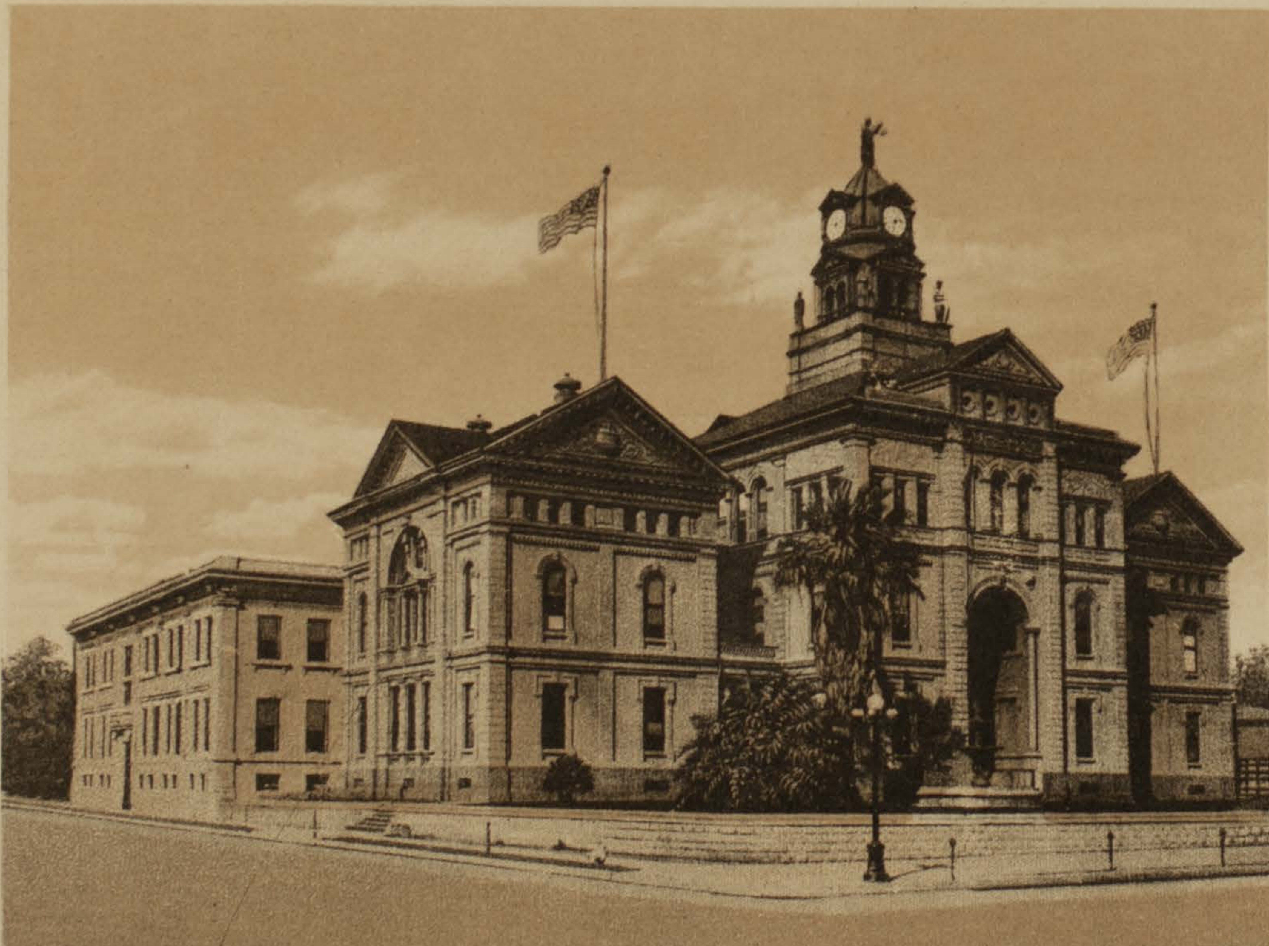
County Court House and Hall of Records.
