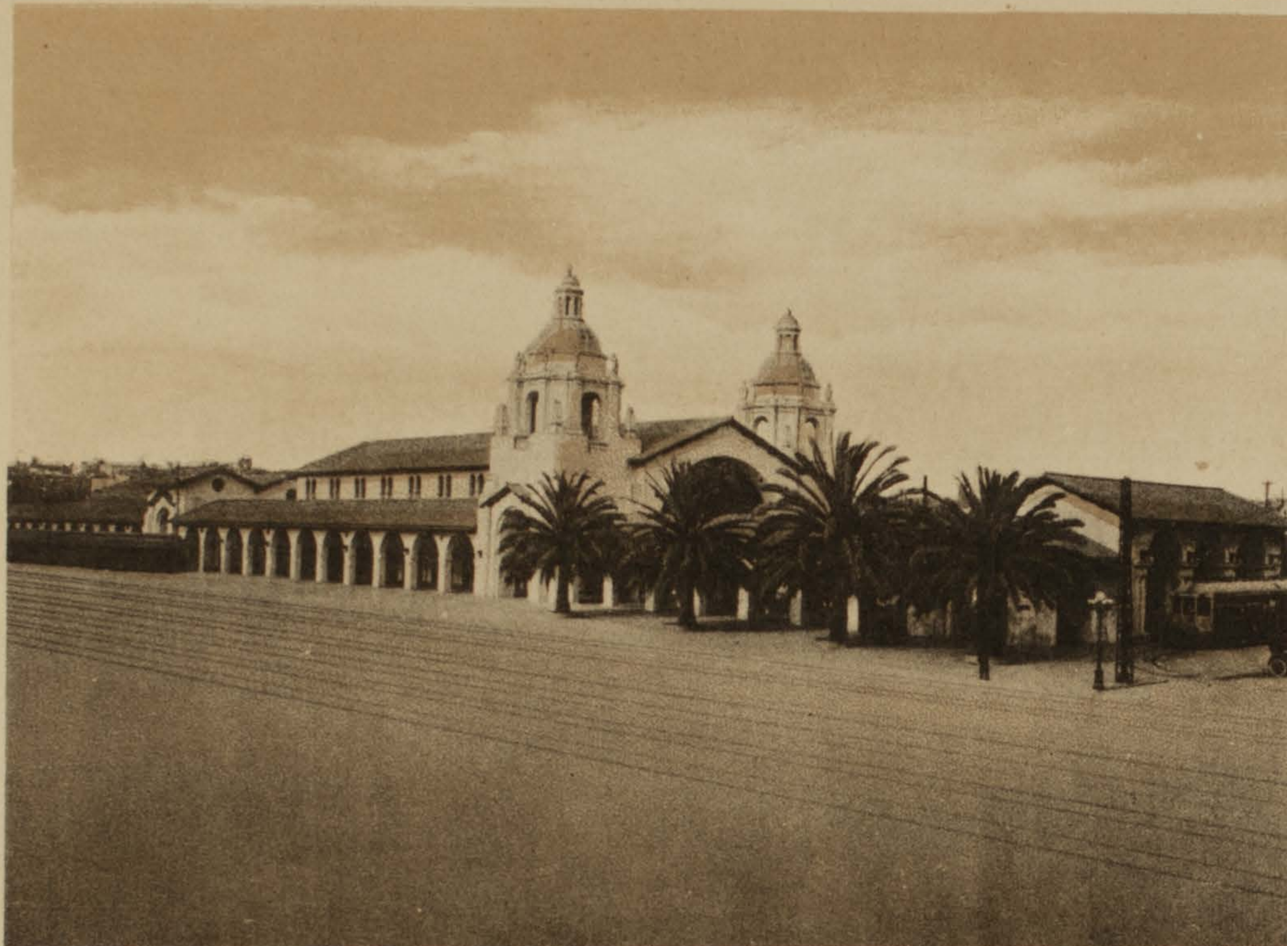
Santa Fe Railroad Depot.
