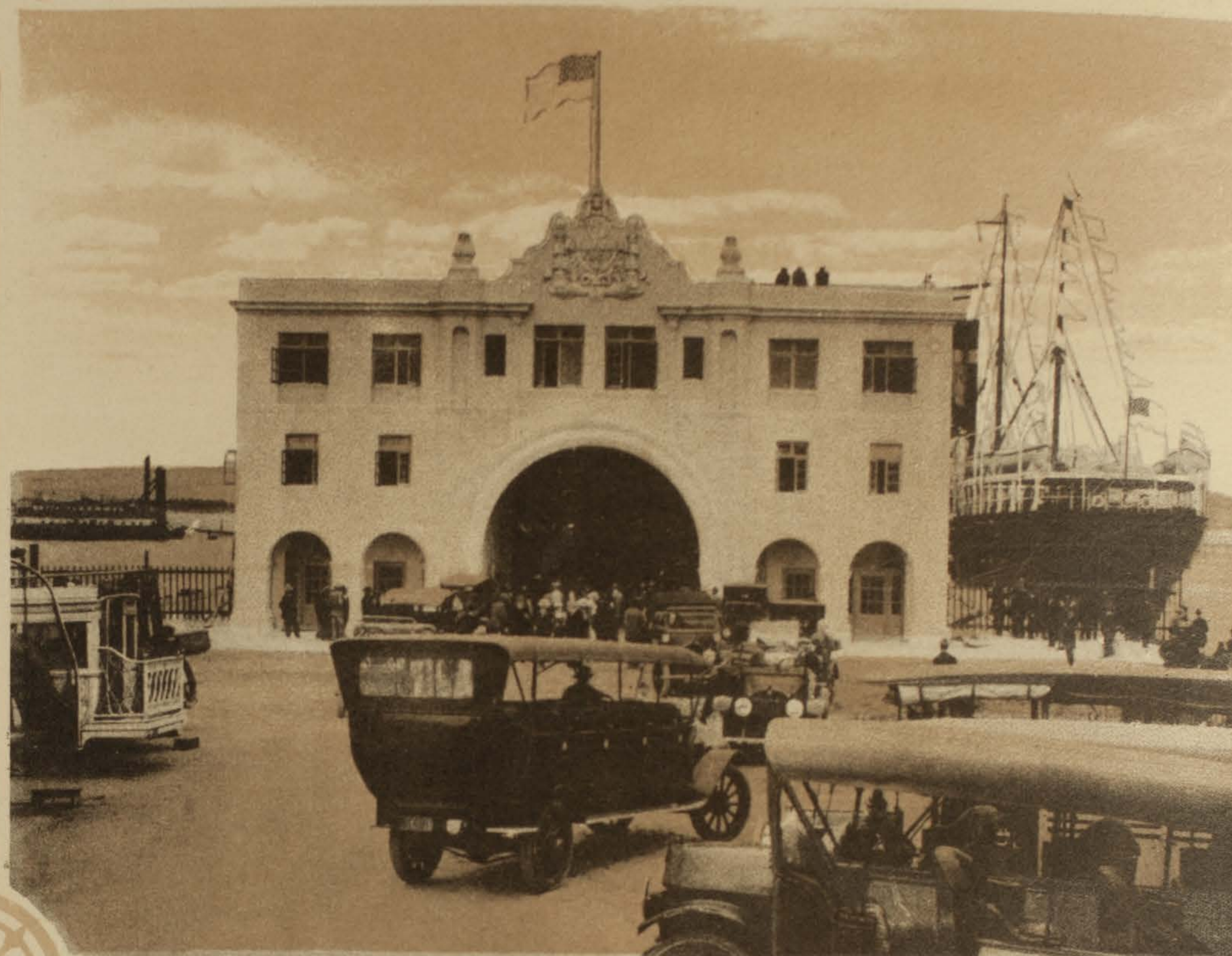
New Municipal Pier.
