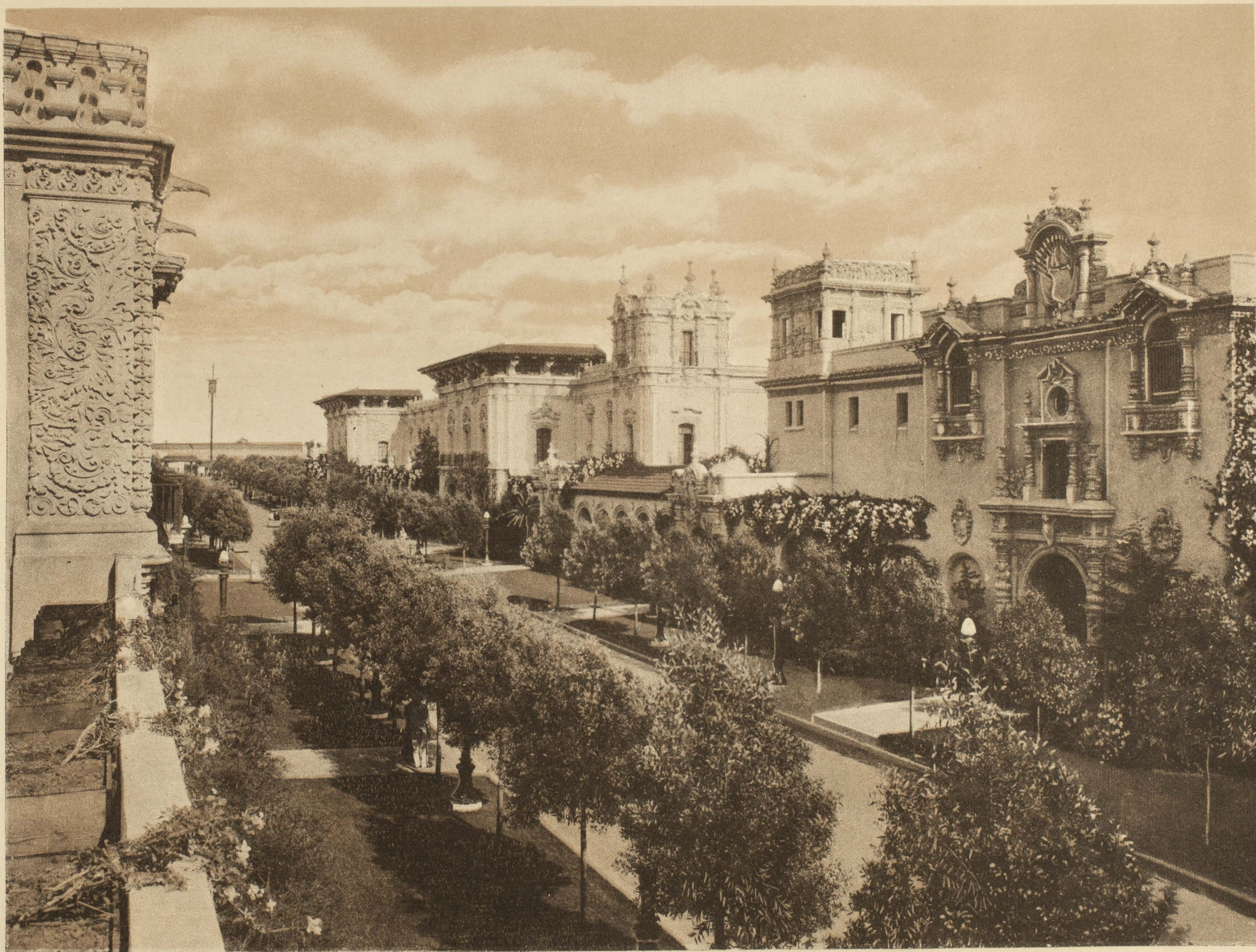
El Prado showing Commerce and Industries Building.
