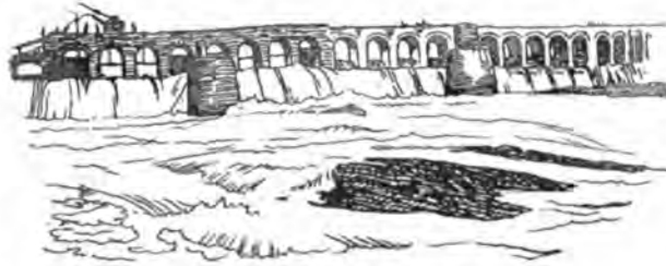
PARTIAL VIEW OF WASTE WEIR OF LAKE FIFE SHOWING THE FLOOD GATES
